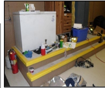
Example of Raising Utilities above Design Flood
