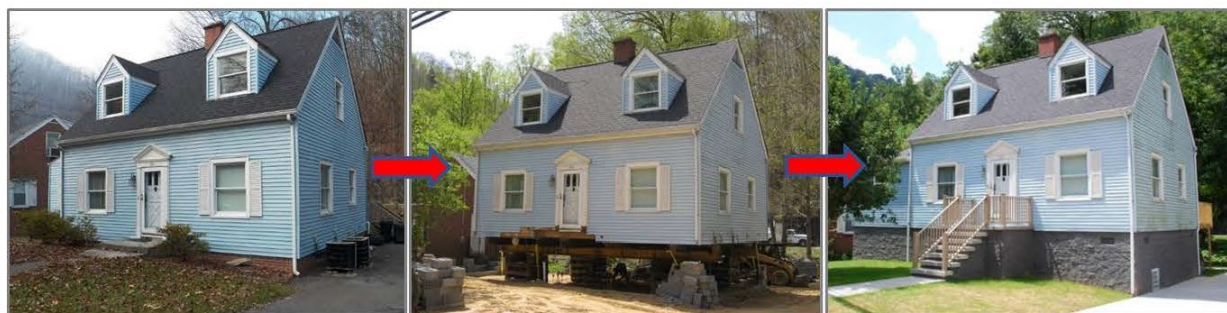
Figure 3-16 Example of Structure Elevation for Flood Risk Management
